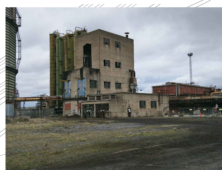
COAL CRUSHING HOUSE
