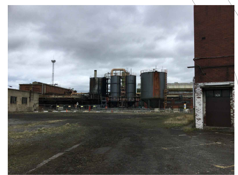
TAR STORAGE TANKS
